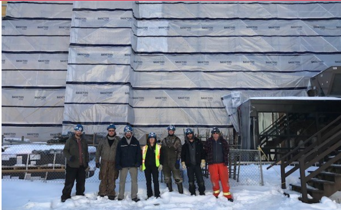
Local 83 Scaffolders from Sancton Access seen above on site with MPL. (left to right) Nate Hale, Jason Cook, Danny Hawley, Karen Bennett, Philip Baxter, Francis Chaisson, Warren Munroe.
