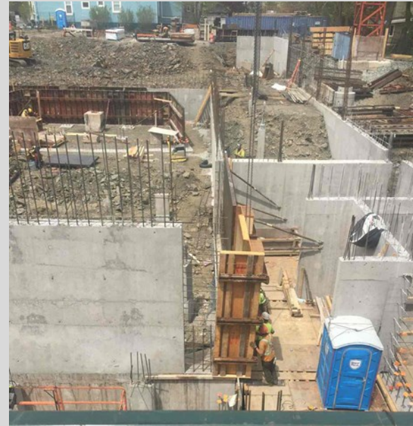
Above: Omega Formwork (Ellis Don), Dalhousie University Arts Center.
