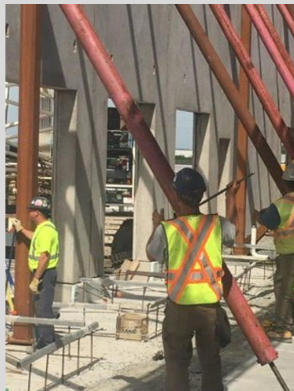
Above: Lindsay Construction, Leons Distribution center, Burnside, NS
