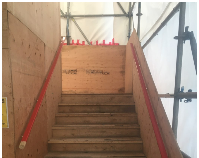
Sancton at Woodside Ferry Terminal. Very rare to see wooden stairs being used on a scaffold, as the public needs to use the scaffold to access the ferry.
